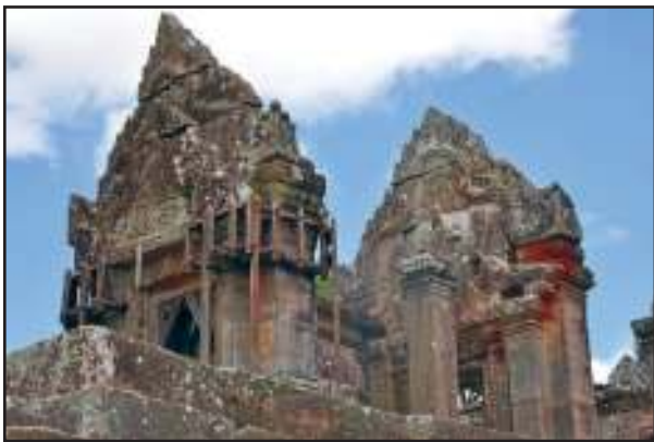
Mandapa under repair
