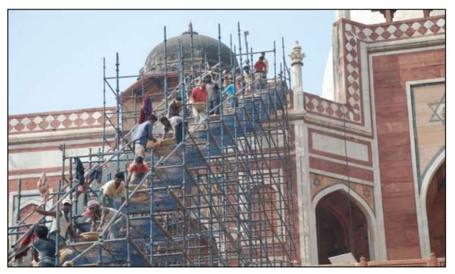
Centuries old building craft traditions were employed in the restoration of Humayun's Tomb wherein modern alterations required to be removed — including 1 million kilos of concrete laid on the roof in the 20th century
