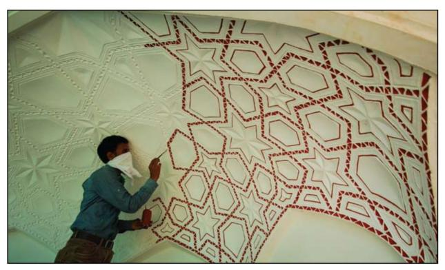
The star shaped patterns adorned the ceilings of the ground level arcade - discovered under cement layers. These patterns were carefully restored on all 68 half-domed arches
