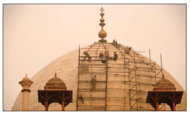
Thousands of stone joints in the dome were required to be carefully filled with traditional lime mortar. The 18 feet tall finial on the dome was also replaced with the original to be displayed at a site museum
